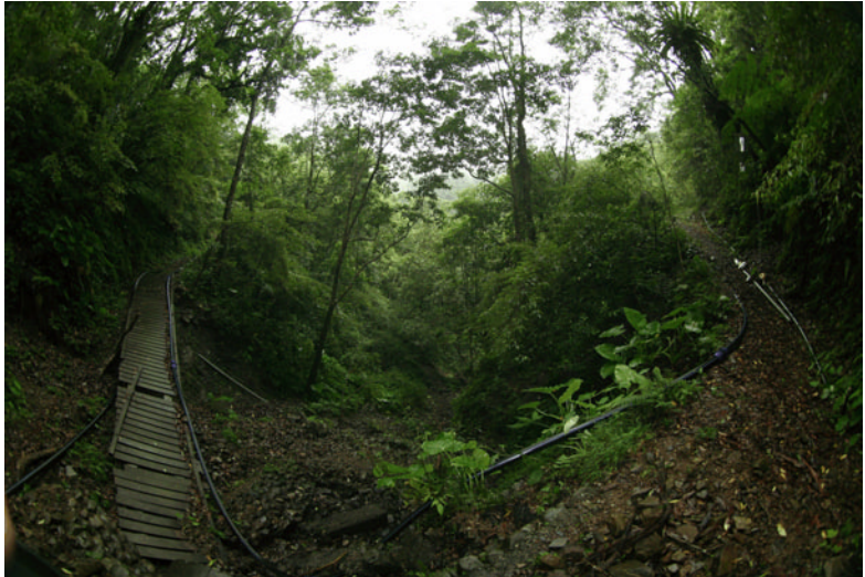
A slightly broken bridge
